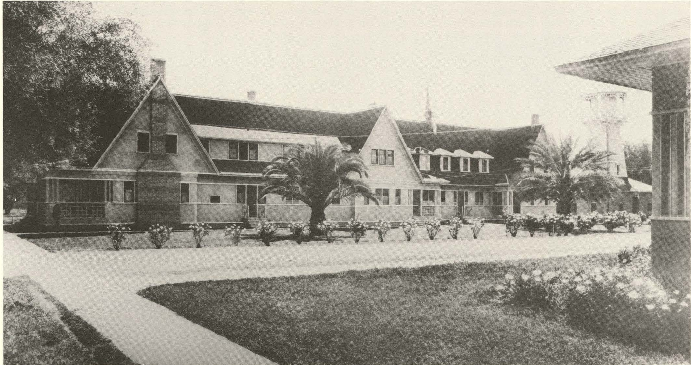
Ingleside Inn, when completed in 1909, was the first resort in the Salt River Valley. The main club house, pictured here, was 150 feet long, finished in grey stucco, and contained dining rooms, living rooms, offices, a kitchen, and a limited number of guest rooms on the second floor. Guest cottages provided the main accommodations, and a corner of one of them is visible on the far right. The Orange Belt and Scottsdale Railroad was to have run by the inn, making it one of the major stops on the line. The entrance to the tree-covered driveway of Ingleside Inn was six-tenths of a mile east of the falls of the Arizona Canal, along what would become Indian School Road. (Arizona Department of Library, Archives and Public Records)
