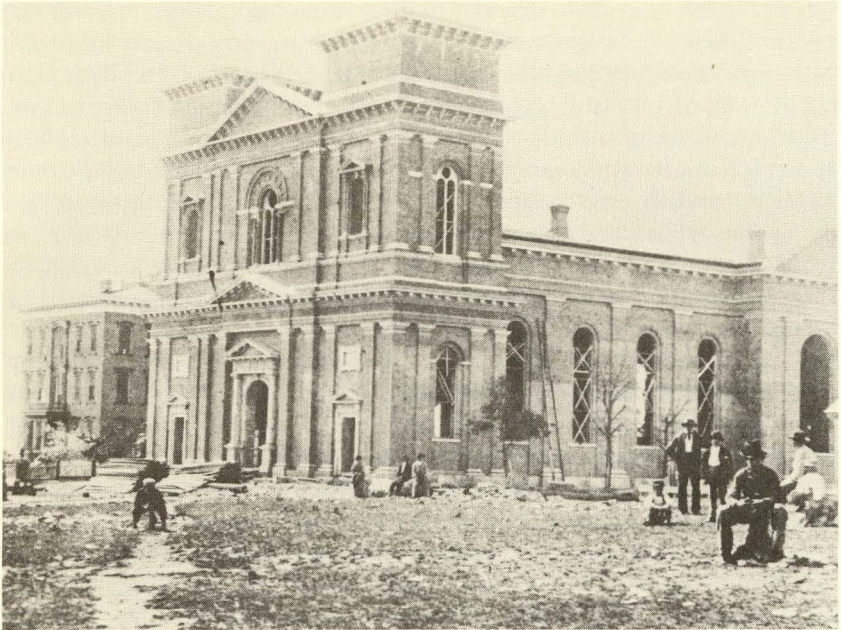
Cathedral of the Immaculate Conception under construction in Leavenworth, 1867. (Kansas State Historical Society)
