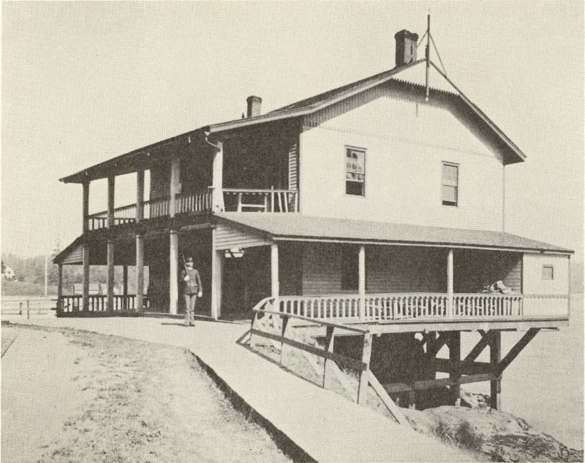
Guard house at Fort Canby. Second story served as the post chapel during Chaplain Scott's tenure there. (Quartermaster General Photograph, National Archives)
